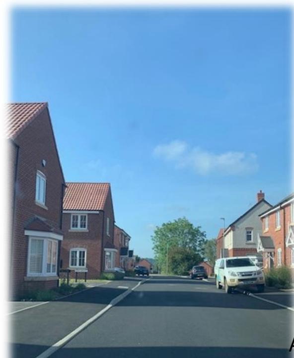
Figure 13: View down the central road running through the development
